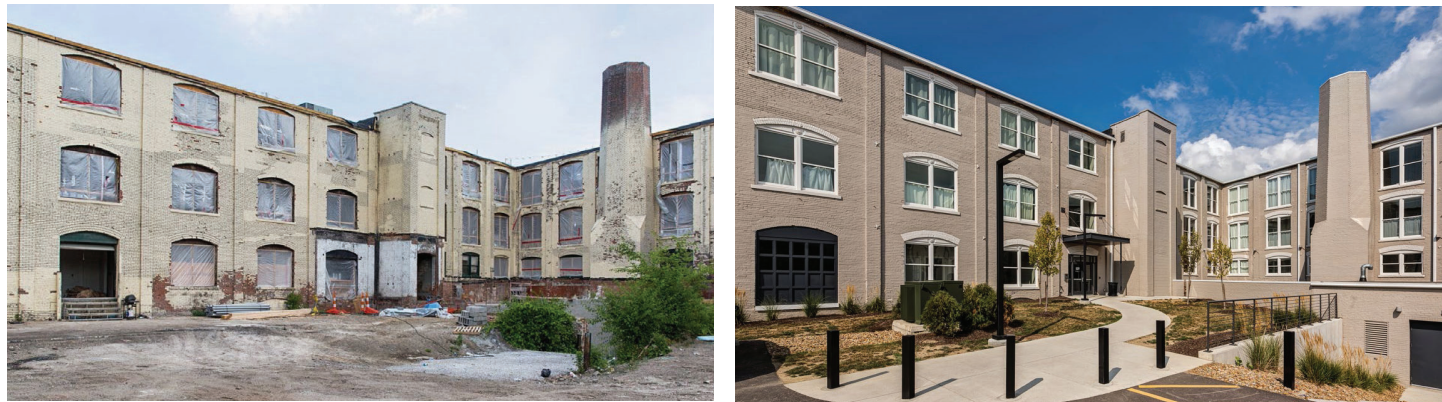
Before and After, The Wagner Awning, Tremont, Completed 2016
