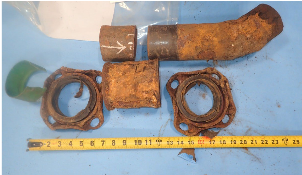
Figure 13: Evidence #2 - south service line coupling near connection to main and elbow segment, and Evidence #6 - south service line, upstream end segment cut for pressure test.
