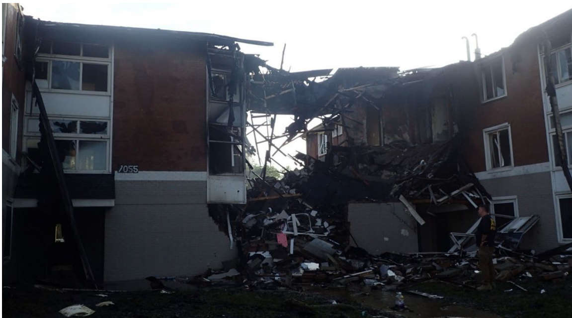
Figure 4: Explosion area viewed from the north, looking south.
