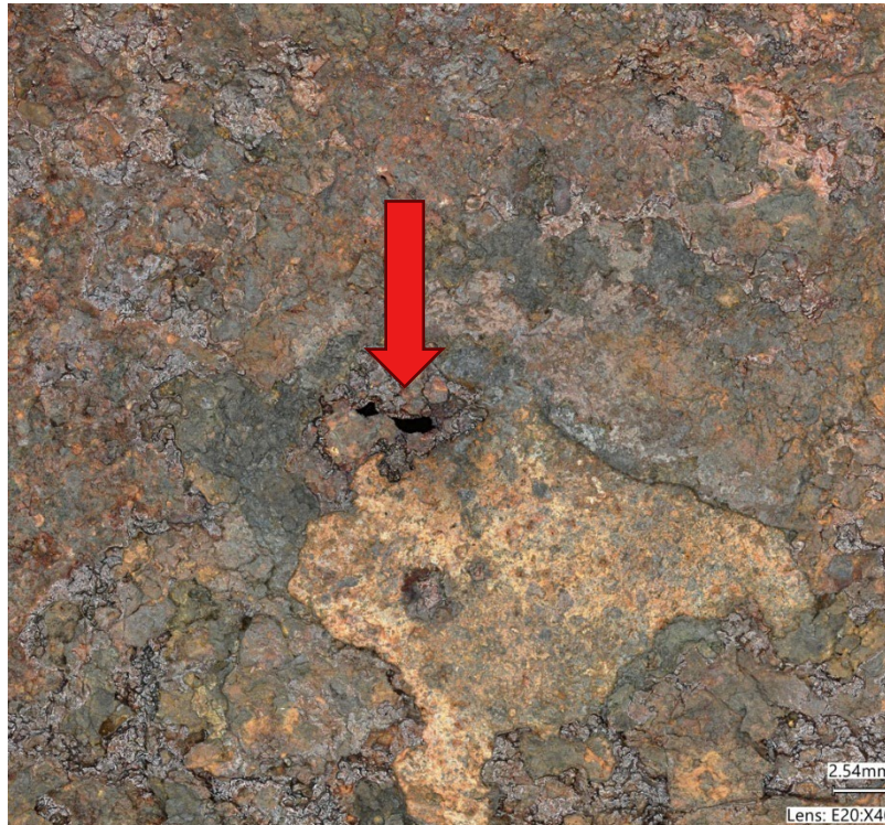
Figure 19: Evidence #3 - pipe exterior surface in area of the leak.
